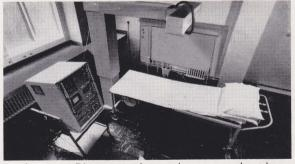
In the new Diasonograph, maximum use has been made of floor space without any sacrifice in the facility of selecting the more difficult scanning planes. The construction of the scanning system and the control cabinet affords considerable **freedom of choice in the layout** of the examination room. Total system weight is 650kg. (Photo courtesy Design Magazine and Philip Sayer)
