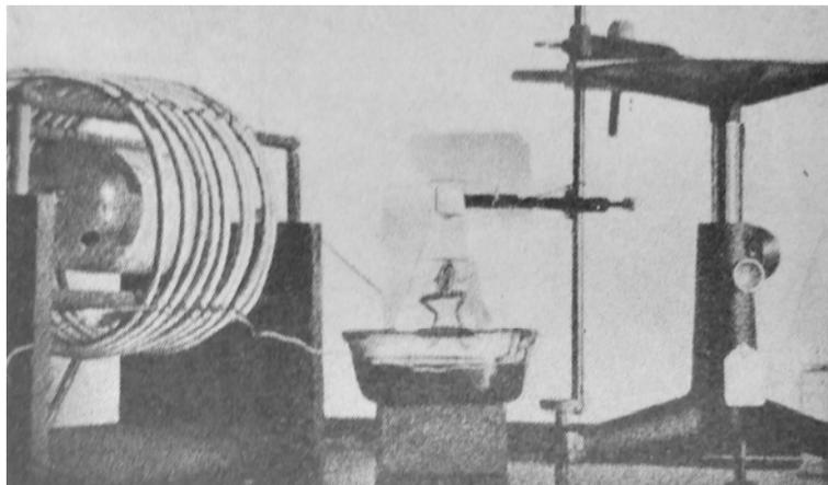
Fig 10. The coil and reaction chamber used by Wood and Loomis in their studies into the physical and biological effects of high-intensity ultrasound. [42]
