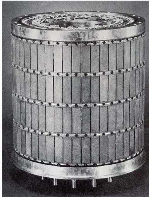
Fig 18. US Navy Scanning Sonar XQHA transducer with rubber cover removed. 1945. [92]
