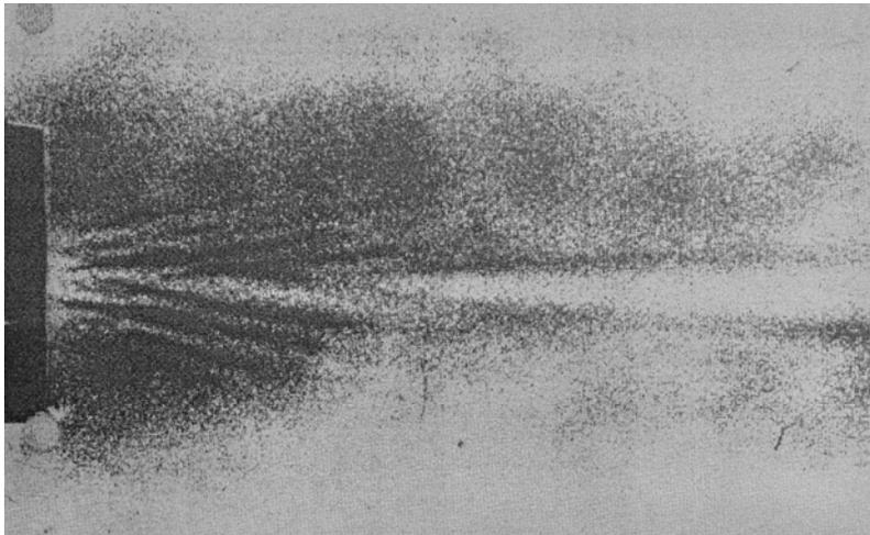
Fig 8. Boyle's dust images of the field of an ultrasound beam from a 178 kHz, 15.3 cm diameter circular source. [31] 1928.
