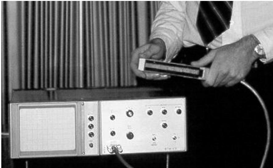
Fig. 35. The popular 61-channel ADR linear array scanner, produced by the Advanced Diagnostic Research Corporation in the USA, in 1973. Photo courtesy of the BMUS Historical Collection.
